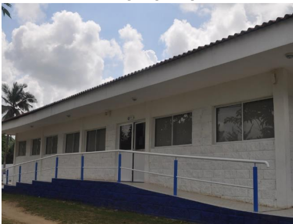
BARANDA SALON MULTIPLE
